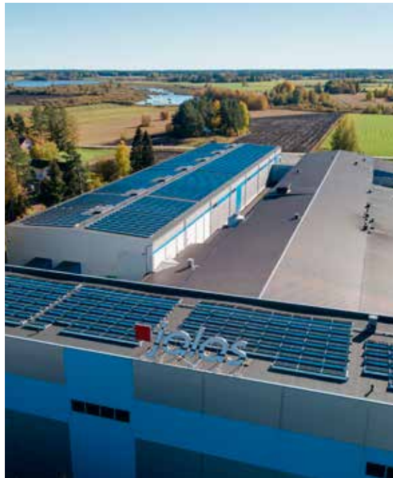
During 2021, we installed a 400+ MWh/year solar panel system in Jokipii, projected to give 20% of the site's annual electricity need.
